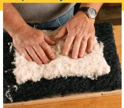
**Start in the middle.** Peel apart some 1-in.-thick cotton batting and place a <sup>1</sup>/<sub>2</sub>-in.-thick piece in the center. Stop 2 in. from the edge.
