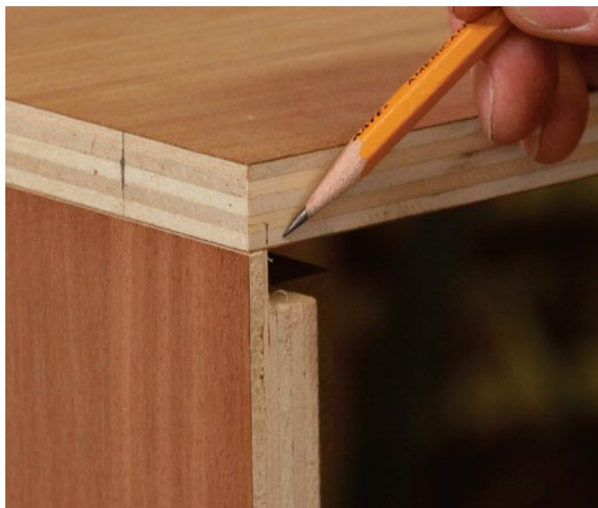
Trim the top. After cutting the mortises in the top and bottom, trim those parts to fit inside the rabbets in the sides.
