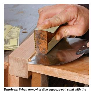
grain using P220-grit sandpaper. Keep the block flat against the work to avoid rounding over an edge. Shield adjacent surfaces with a wide drywall knife.
