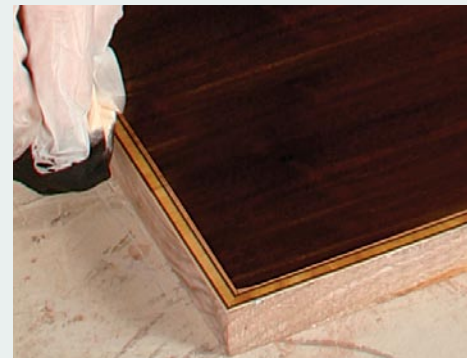
Seal the inlay. Apply several light coats of lacquer to the unmasked banding (left). Then wipe or brush on a dye or stain that won't dissolve the sealer (above).
