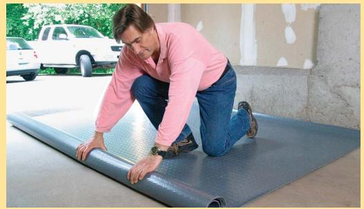
Cover a large surface area in no time. The large, heavy rolls are easy to install once in position. Wait for warm weather, as the PVC material is more pliable and easier to unroll above 60°F.
