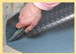
Trim with a utility knife. Before trimming the excess material, allow it to relax at the base of the wall.
