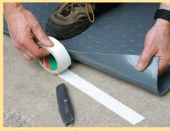
Hold down edges with tape. When taping the edges, use indoor/outdoor double-faced tape.
