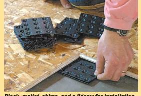
Block, mallet, shims, and a jigsaw for installation. Protect the tongue-and-groove edge with a block when knocking the tiles into place with a mallet (left). Leveling spacers are easy to position and compensate for any unevenness in the concrete floor (above). With the tiles on a stable support, cut them to size with a jigsaw.
