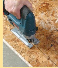
tongue-and-groove product was created as a base for carpet, vinyl tile, or engineered hardwood flooring, but it may be used as is. The color of DRIcore is a natural-wood tone, and the surface can be painted. A mallet and a jigsaw are all the tools required for installation.
