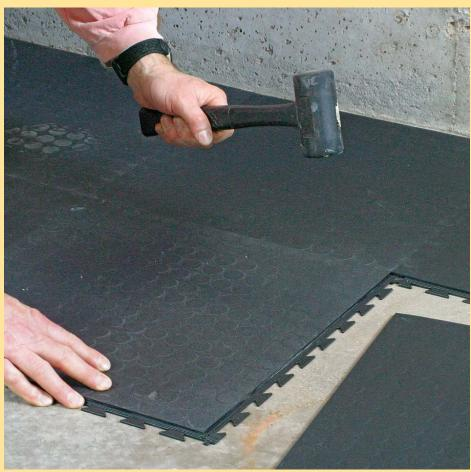
The tight interlocking tabs are joined easily with a mallet. Knock the interlocking edges into place with a rubber mallet for a snug, flush seam.
