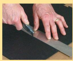
Trim the tiles with a utility knife and a straightedge. PVC tiles are thin enough to be cut to size with a standard utility knife.
