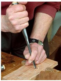
Chop out the rest. Insert one corner of the arm stock to test the width of the mortise.
