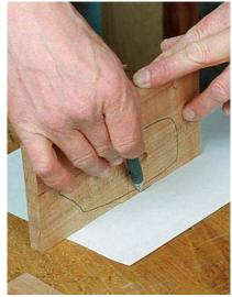
More fun with paper. To make an accurate angled mortise, start by tracing the thickness of the fence onto paper.
