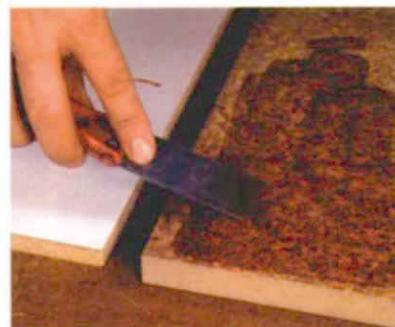
*Work mixture into the grain. Apply it in one direction, and then work it into pores crosswise. Try to create a smooth surface.*
