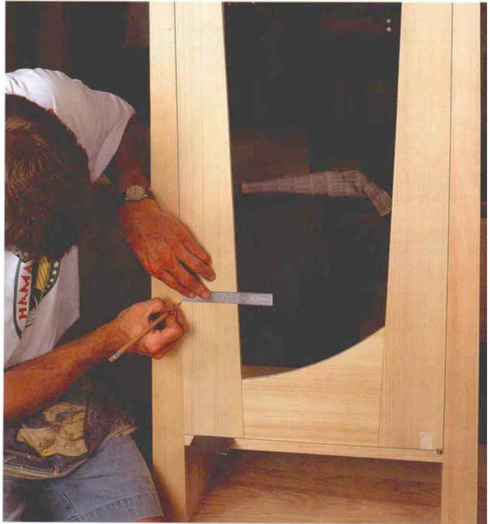
*Good installation starts with a good fit. The author uses plastic laminate shims to set a narrow, reveal between the door and the carcass. Then he marks how much to trim off the door.*
