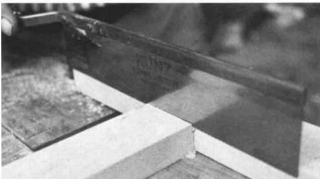
assembled, make a clean saw cut along the shoulder line, making sure not to cut into the mortised piece at all. Do the same for the other shoulder. Don't saw quite completely to the tenon. Instead, finish the cuts with a chisel after the joint is disassembled. If you're making a frame and notice one of
