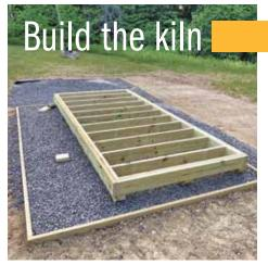
**A firm and dry foundation.** The kiln's deck is framed with 2x6s on 12-in. centers. It rests on 4x4 skids running lengthwise and a 6-in. bed of  $\frac{1}{2}$ -in. stone for drainage.
