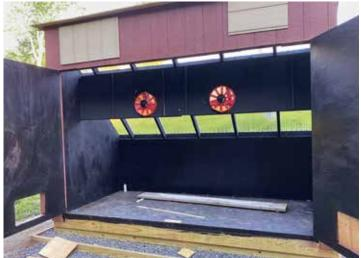
**Different paint jobs outside and in.** The exterior surfaces, all T-111 paneling, are painted with ordinary house paint. But inside, the floor, walls, and doors, all paneled with ½-in. CDX plywood, get a rubberized black coating that acts as both a moisture barrier to protect the framing and a passive solar heat sink.
