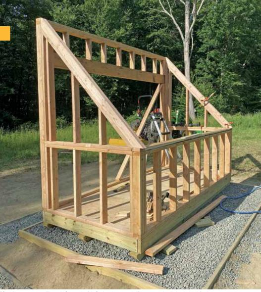
**Simple structure.** Though framed with 2x lumber much like a standard shed, the kiln has some members doubled up for rigidity.
