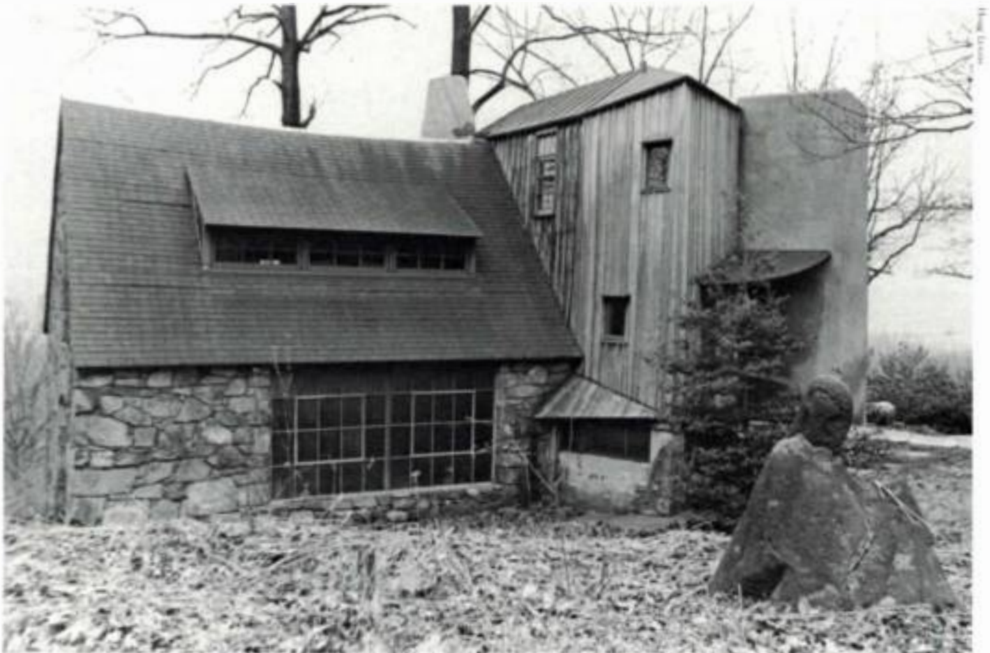
Esherick began work on his studio in 1926. It later became his home, and he continued to modify and add to it throughout his lifetime. The lower windows look into the main workshop (now a sculpture showroom), the upper windows into Esherick's bedroom and library. The tall wooden section contains a dining area on the first floor (with a deck attached) and a bedroom above. Esherick had always wanted a silo and in 1966 added the concrete one at right to house a kitchen and a dressing room. He directed two masons with buckets of pigmented cement to fresco the exterior in an abstract pattern inspired by the autumn colors of the landscape.
