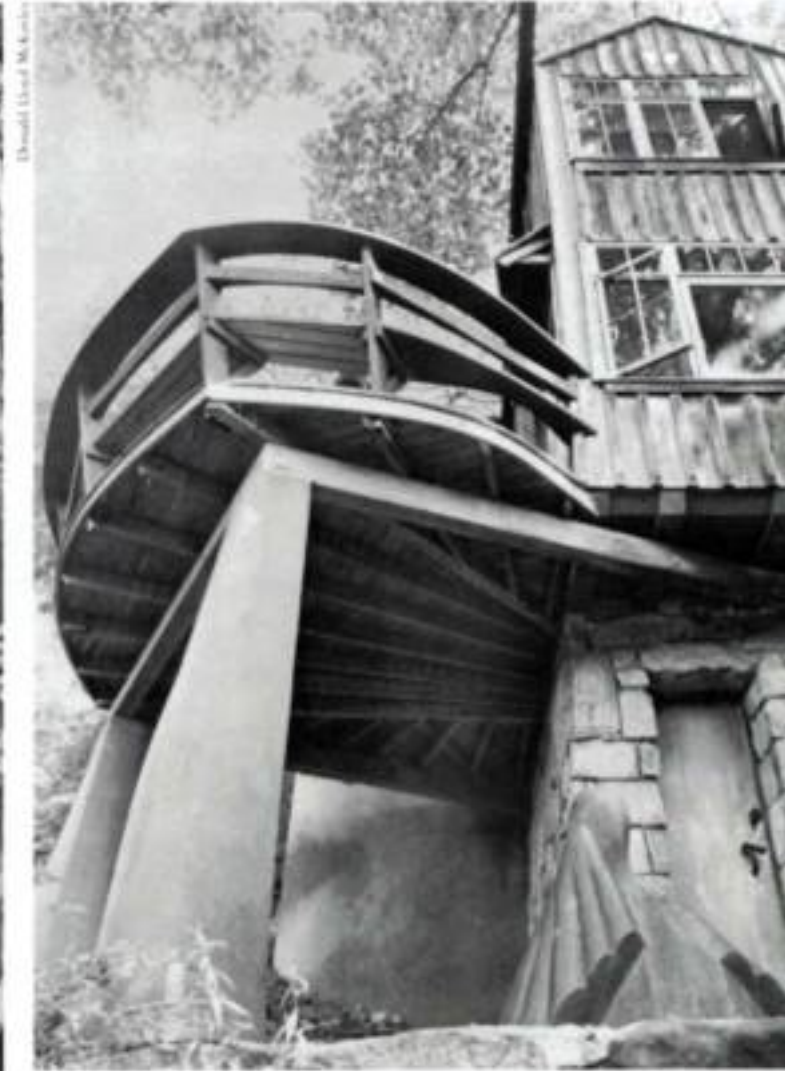
The south face of the Esherick studio and home includes the door that opens onto the coat room (shown behind the staircase, p. 54). Above is the dining area, and above that a bedroom. The foundation is limestone, the siding roughsawn oak, and the deck cedar and fir, supported by stone and plastered pillars.
