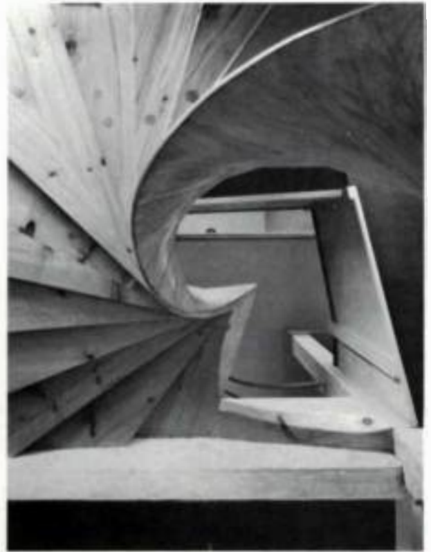
Stairs, left and above (seen from below), designed and built for the front hall of the Bok house (1935) from solid white pine beams.
