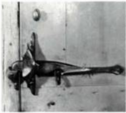
Carved rosewood latch (1926) inside the front door is typical of the detail work in Esberick's studio. He designed and made everything from lamps and switchplates to radiator covers, all to this standard.
