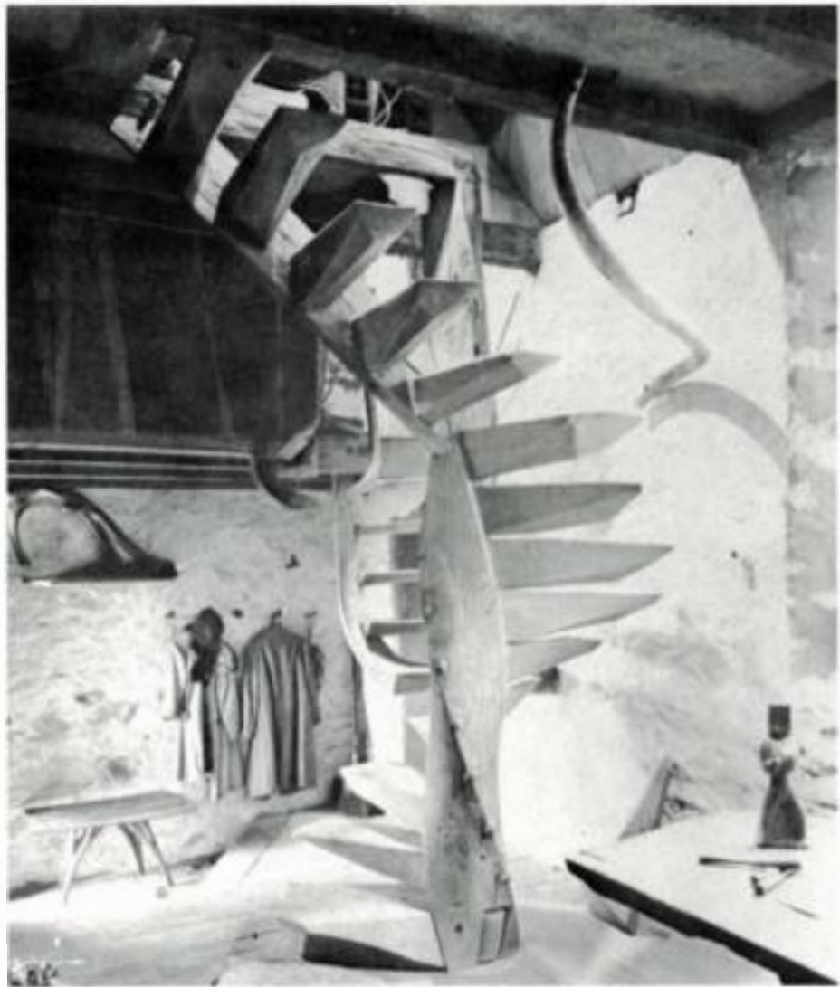
Red oak spiral staircase, made in 1930, connects the main floor, the dining area and Esberick's bedroom in the loft (right). Despite its unorthodox shape and lack of a continuous handrail, feet and hands travel effortlessly upon it—a tribute to its cunning construction. The steps are tenoned into the massive post and drawn up with 8-in. bolts through nuts set into the tenon.
