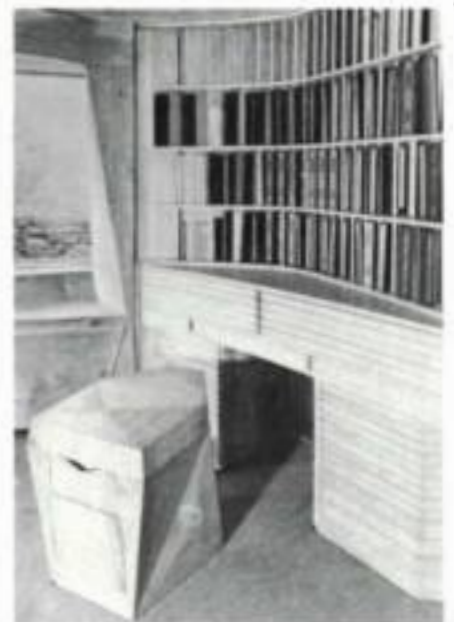
Library fireplace and music-room doorway of the Bok house, above. The arches over fireplace and door were built in 1936 of white oak. The music-room fireplace in the background is plaster and the ceiling is white pine boards joined with full-length tongue and grooves. The curved storage unit for phonograph records and sheet music, right, made of cherry, is built into a corner. The angle of the partitions is varied to utilize the depth of the corner and to provide easy access to all the albums. The separate unit is a radio-phonograph cabinet. The window, sculpted to resemble a curtain blowing open, reflects the spirit of playfulness Esberick brought to much of his work. In the Bok's dining room, the fireplace mantel (1935), above right, is solid chestnut oak with a stone hearth, surrounded by a copper arch.
