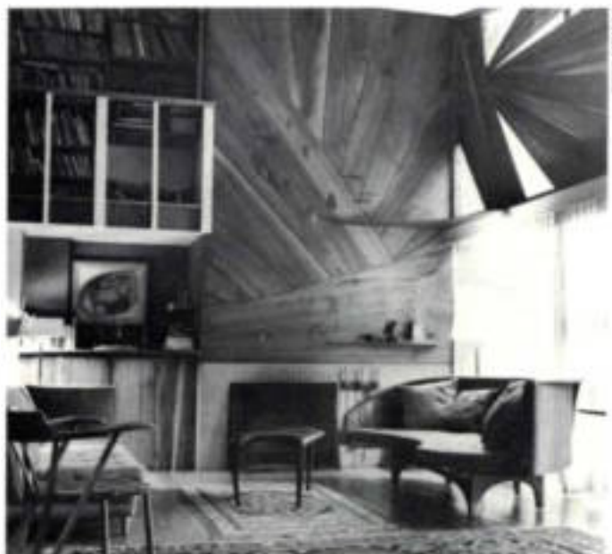
During the 1960s Esherick did extensive work for Lawrence and Alice Seiver of Villanova, Pa. Window and fireplace paneling in their living room is tulip poplar; construction is shown below. Esherick also made the shelving and curved paneled sofa.
