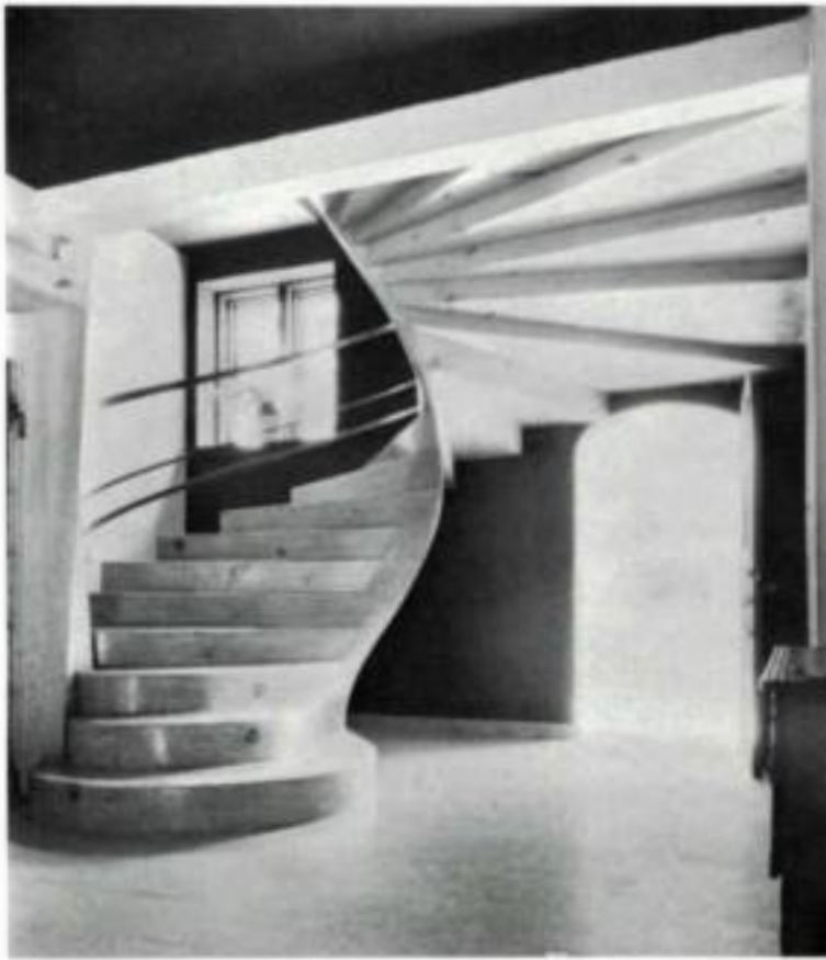
Stairs, left and above (seen from below), designed and built for the front hall of the Bok house (1935) from solid white pine beams.
