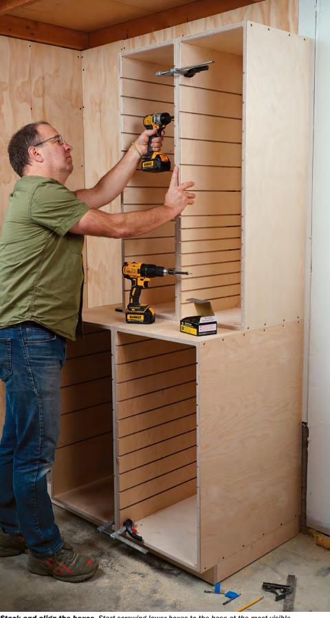
**Stack and align the boxes.** Start screwing lower boxes to the base at the most visible end, making sure they are flush with the base and each other. Align their front edges carefully as you move down the line. Then screw the upper boxes together. Wait until the end to connect the upper and lower boxes, then screw the whole unit to the wall. Let the base float outward if necessary; if there's a gap at the top, shim it before driving screws.
