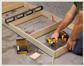
How to level the base. Start by leveling the back edge from end to end, placing shims underneath where needed. Then use more shims to level the base front to back. When it's level in every direction, screw plywood feet inside the base to lock it at that level and support the heavy cabinets. Don't attach the feet to the floor.
