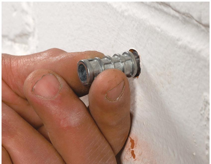
When you want to attach with screws or lag screws, use lead sleeve anchors. These old-style Everbilt soft lead lag sleeves (2) are studded with projections and built in two loosely connected halves, allowing them to expand and shift in shape to conform to a predrilled hole when the screw is driven home.
