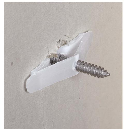
**Squeeze the wings and hammer the anchor home.** After predrilling, fold the anchor's wings together and push it into the hole, then tap it home with a hammer until the flange is flush with the wall surface. With the anchor in place, use the supplied plastic pusher to pop open the wings. Then drive the screw.
