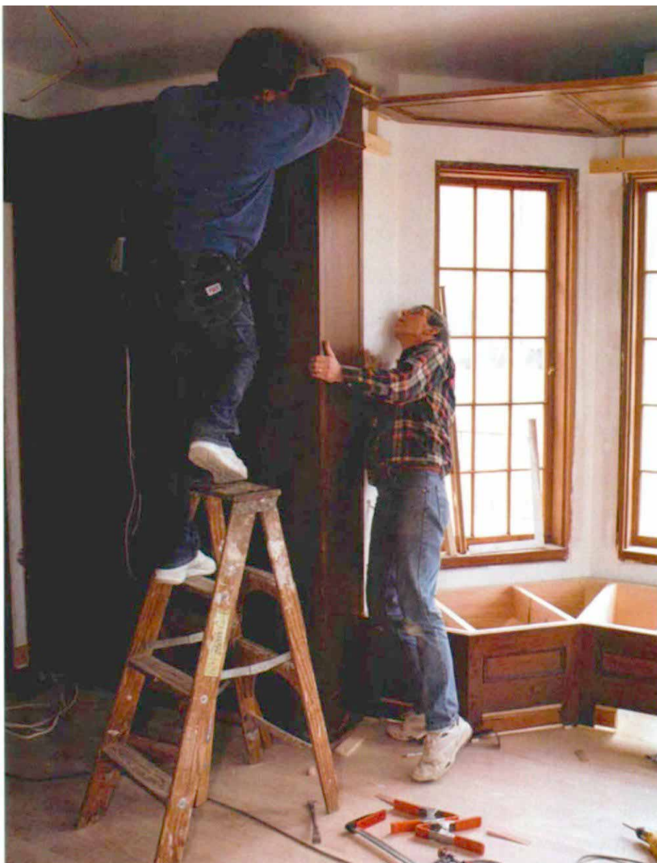
Installing the case work—Job-site conditions usually require shims to make cases level and plumb (above). The result is a beautiful library and plenty of sawdust back at the shop (right).
