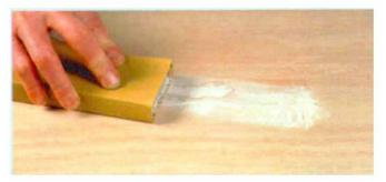
**3.** Sand putty before removing tape. Once the putty has dried, he uses a sanding block to remove the excess.
