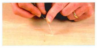
**2.** Cut and remove a football-shaped patch. With a sharp razor, he cuts an irregular shape around the hole to be repaired. He will fill that and the other hole with latex putty.
