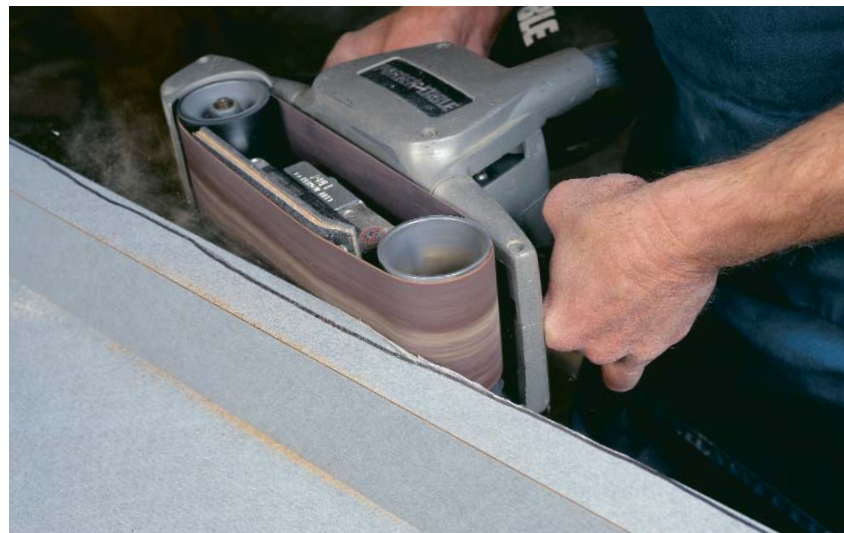
Scribe to fit. By using the front wheel of the belt sander, you can cut into tightly scribed areas, like this plastic laminate backsplash. A saw would likely chip out this material, and a block plane would dull very quickly.
