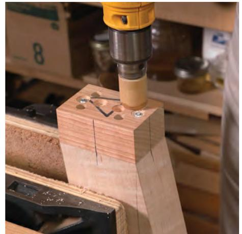
**Holes for the rod.** Using a handheld drill with a bubble in the handle and a shopmade depth stop, Coleman cuts the four holes for the threaded rod. He uses a brad-point bit sized to make a hole the rod will slide into easily.
