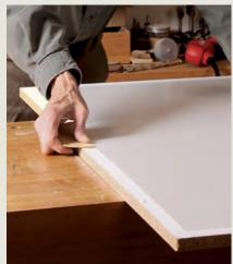
Attach the top. The top gets glued and clamped to the frame. If you are using a sheet with melamine on both sides, make sure to scuff-sand where the glue will be applied. Because there's no way to apply clamp pressure at the center of the tabletop, Becksvoort glues a cleat to the supports, and then predrills and screws through the cleats into the underside of the top.
