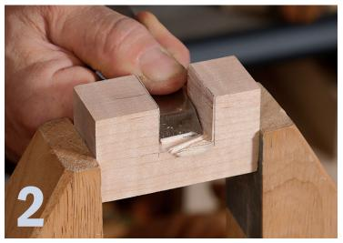
**Pare the floor.** Use a wide chisel to flatten the bottom of the notch (above). Check with a square to be sure you pare the bottom of the notch 90° to the sides of the jig (right).
