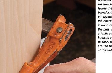
Transfer with an awl. Miller favors the awl for transferring the pin layout to the tail board (left), as it won't cut into the pins the way a knife can. Then he uses a knife to carry the lines around the corners of the tail board.
