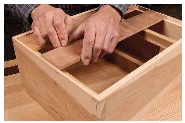
**Cut and test.** Use a tablesaw or miter saw to crosscut the board close to the mark, and then try the fit. When it's perfect, crosscut other backboards with the same machine setting.
