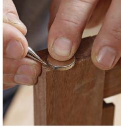
Mark the mortise wall. For strength, leave 1/6 in. of material between the mortise and the inside face of the door (left). Center the 3/4-in. magnet on your first line to find the ends of the mortise (right). Add  $\frac{1}{32}$  in. on each end ( $\frac{1}{16}$  in. overall) to give the magnet some wiggle room.
