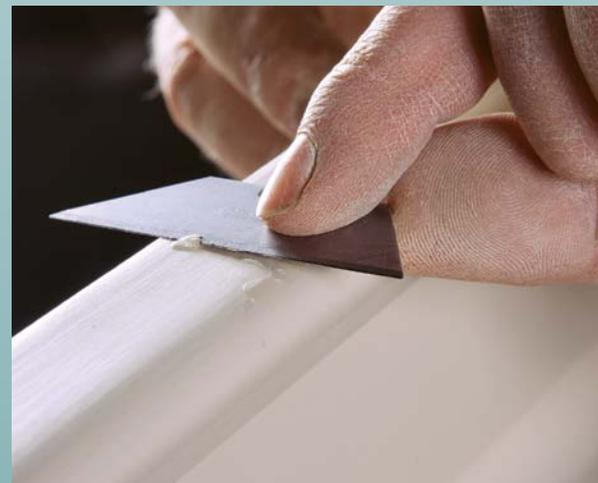
**Deal with drips.** If you can't catch a drip or run immediately, don't wipe the sticky surface. Let it dry, then shave it flush with a sharp knife. Clarke uses a utility blade.
