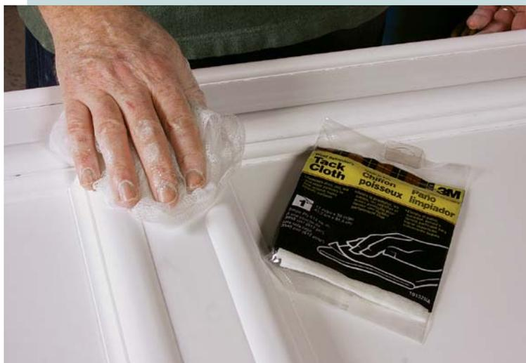
**Remove all dust.** After vacuuming the surface, lightly wipe it with a tack cloth to remove any remaining residue.
