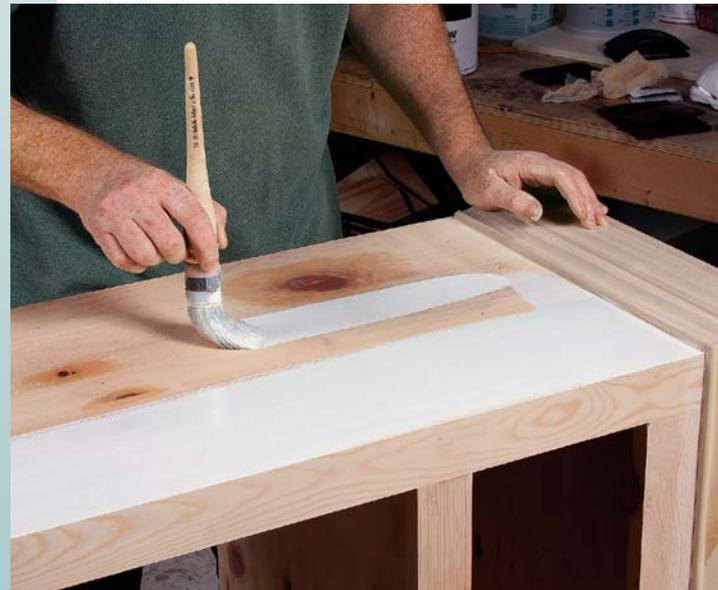
**Best technique for flat areas: Unload, then spread.** Load the brush and then lay down a thick strip of finish away from the edges (left). Then come back and spread the finish out on both sides of the strip (center). After reloading the brush, land it an inch or two from the wet area (right). Now it, too, can be spread out on both sides and will not create a ridge of excess finish.
