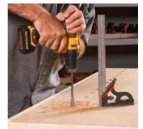
Install the vise. Sighting along an upright square (above) helps in drilling a straight dog hole. When you attach the vise (right), add a spacer block to keep the jaws even with the tabletop.
