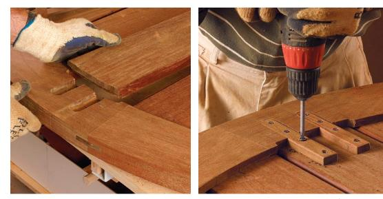
**Cleats support the last board.** Fitting into channels routed in the ring, two cleats made from ipé scraps are screwed home.
