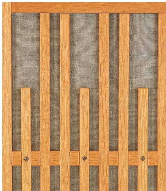
A unifying theme. Latticework is used on all of the cabinet doors. Some intersecting members are pinned using brass, colored an antique brown.
