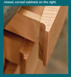
I-beam—it has a plywood back that acts as a stiffening spine and open, solid cherry shelves on both sides. To make this improbable arrangement work, I drilled right through the exterior wall and bolted into the shelving unit from outside.
