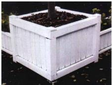
Paint can't overcome poor design. This unlined, wood planter box is destined to fail because the moist soil holds water against the wood, allowing it to seep into the joints, and these joints aren't designed to drain water. The unprotected end grain of the feet also wicks up water from the puddles in which the planter stands.
