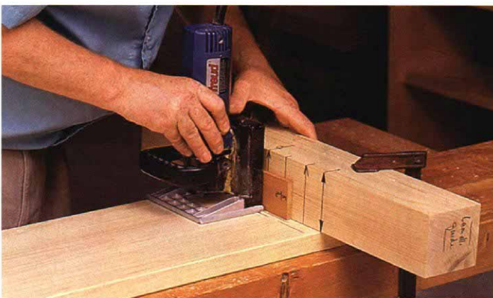
To slot the faces of the uprights, square a line that locates one edge of the fixed shelf. Clamp the 4x4 gauge right on the line, and with the machine vertical, run the first row of slots. Then place a spacer— \frac{3}{16} in. thick in this example—between the machine's base and the 4x4 to cut the second row of slots.
