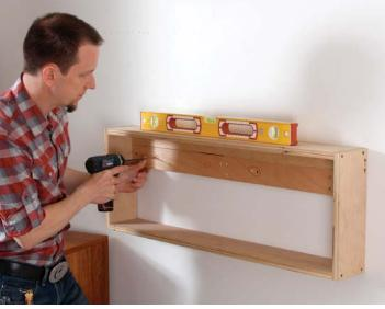
**Hang man.** To help arrange and hang the boxes on the wall, Chaffin uses a backless box. The box makes it easier to lay out the 3-D shelves and install the French cleats that they mount to.
