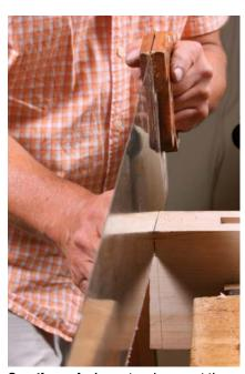
**Saw the ends.** Lay out and crosscut the angled ends. Smooth them with a handplane, and plane the curve into the top.
