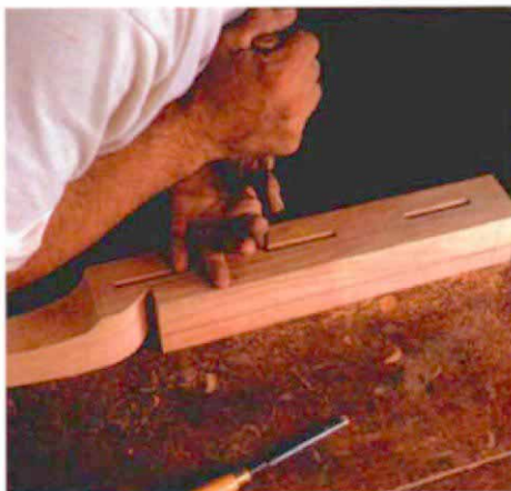
After the router, use a chisel to pare and square the mortises to the scribed lines.
