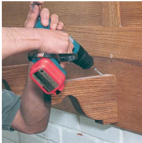
A screw locks the bracket. After the skirt is tied to the wall, a screw is driven at 45° to hold the bracket permanently in place.
