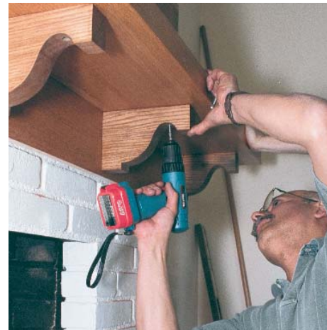
Shelf is attached from underneath. The shelf goes onto the brackets, and an inconspicuously placed screw keeps it there.
