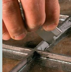
**Apply the glazing.** Use a flat-bladed knife to apply putty along the edges of each pane and draw it onto the muntin at an angle. Then use a single-edge razor blade to smooth the glazing. Don't wait too long to do this, because acrylic putty sets up relatively quickly. Once the glazing sets up a bit, use the razor to remove the excess from the glass and muntins.
