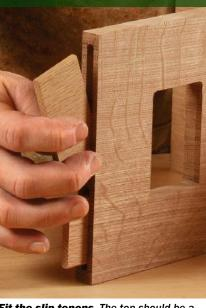
**Fit the slip tenons.** The top should be a close fit, but leave the bottom tenon a bit narrow to allow for wood movement.
