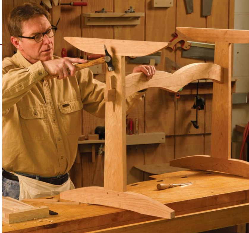
Tap the wedges home. When the wedges are tightly driven, they pull the tenon shoulders firmly against the post for an assembly that won't budge.
