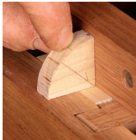
Check the radius. Make a template that matches the column's radius, but with an extra 1/8-in. straight section at each end.
