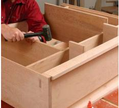
**Long sliding dovetails with no binding.** The trick is to slide in the dividers from the back almost all the way without glue, leaving about 2 in. exposed, and then apply glue to that exposed end and into the slot at the front. Now you can drive the divider home with a mallet.
