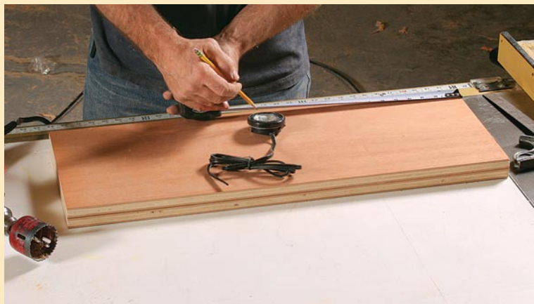
Layout for a recessed light. Casey starts by marking the shelf bottom for the location of the fixture.
