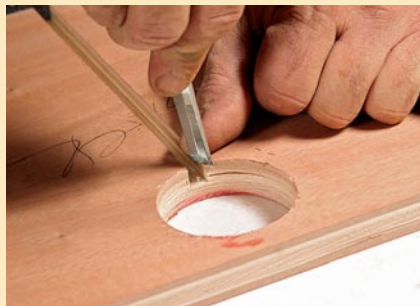
A dado creates a channel for the wiring. Use a chisel to soften the transitions and prevent sharp corners from damaging the wire.
