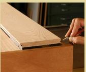
Start in the middle. Space the slats about ½6 in. apart. Rip the outer boards to fit. Nail or screw the outer slats along the edge. Use two nails in each middle slat, about ¾ in. from each edge.
