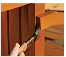
Apply the primer. Once the two-part epoxy is combined, you have about 20 minutes to apply it generously to the surface, letting it saturate the wood. Pay attention to the end grain as this is where weather damage is most likely. Re-coat these areas as the epoxy is absorbed into the wood.
