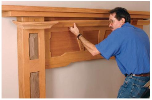
**Attach the finished molding.** When the molding is assembled, slide it onto the mantelpiece and secure it to the shelf with 16- or 18-ga. finish nails.
