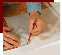
Trace the area to be patched. Draw the perimeter with a wavy line, and then make a Masonite template of that shape.
