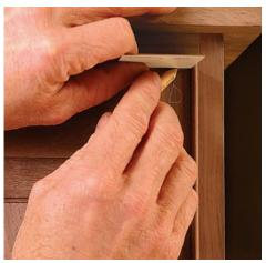
2. Mark the gap at the top. Hold a shim against the top of the case opening and mark the trim line at each top corner of the door.
