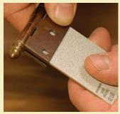
Speetjens uses shims that match the gap between the hinge leaves to create gaps of even thickness around all four sides of the door.
