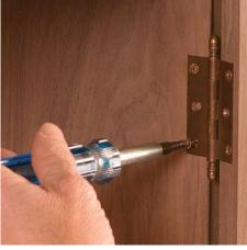
**2.** Hang the door before final trimming. Work carefully to be sure each hinge leaf is set exactly flush with the surface.
