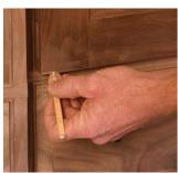
2. Measure the gap and mark the corner. With a few thin shims, measure the thickness of the gap on the hinge side of the door. Then mark the corner of the bottom edge to be tapered.
