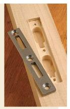
Make room for the clips. The strike plate is recessed into the post. In addition, deeper mortises are required to accommodate the two clips.
