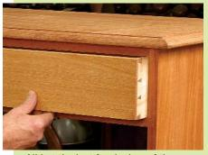
All but the last few inches of the drawer should slide in easily at this point. Level the dovetails at the front of the drawer box and continue planing those areas until you achieve a 1/32-in. gap at each end. Also, touch up the top edge for the same gap.
