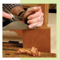
Plane one end to fit the case (above). Then set the drawer front in the case and mark the other end for length at both the top and bottom edges (right). Aim for a snug fit at this point in the process.
