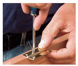
Drive in one steel screw. This leaves two hole locations unused to allow the hinge to be adjusted in or out later. Use a steel screw to avoid damaging your softer brass ones.
