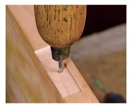
Mark for the center screw. Offset this location slightly toward the back of the mortise to draw the hinge tightly into place.
