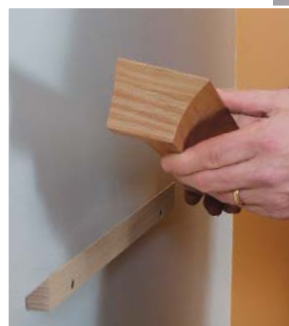
A French cleat bears the weight. The base engages with the wall cleat, and the cabinet sits atop the base. The case requires only a single screw at the top to hold it securely to the wall.
