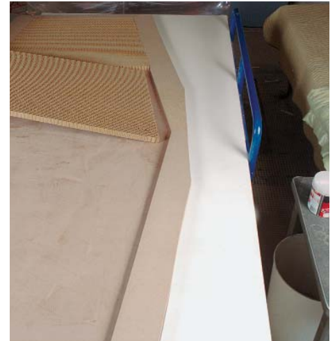
Work from the bottom up. After applying glue to the bottom skin, place the MDF frame and the honeycomb material in place. Fasten the frame to the skin with screws.
