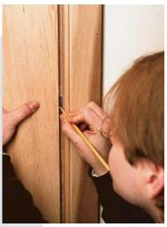
Mark once, cut once. A nickel spacer on the top of the stile and two wedges on the floor hold the stile steady. A centerline is marked alongside the strike plate (above). Laying out the hinge locations with a striking knife (left) is easy work with the stile clamped to the hinges.
