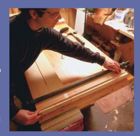
Then holding the bevel tightly against the hinge-side jamb, swing the bevel out across the floor in the angle the door will swing. Any lumps or humps in the floor that will prevent the door from swinging fully open will show up immediately.
