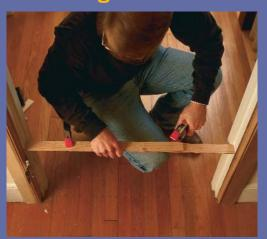
When it comes to fitting parts precisely in trim carpentry and cabinet work, a tape measure is about as useful as a baseball bat in a billiard game. A tape measure has all those spaces between the gradations, and in the real world, things seldom fall right on the mark. So you wind up rounding off to the nearest one-sixteenth.
