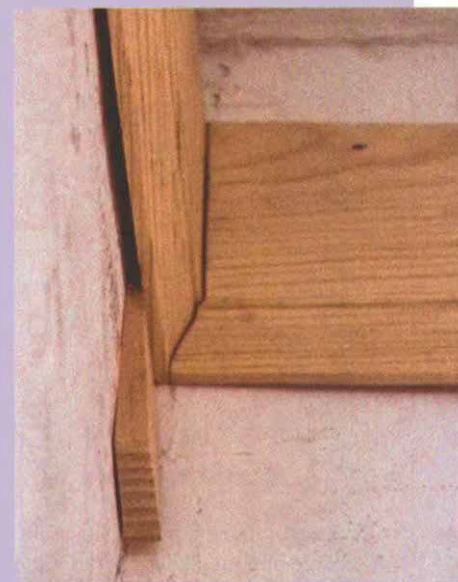
Installed and shimmed
