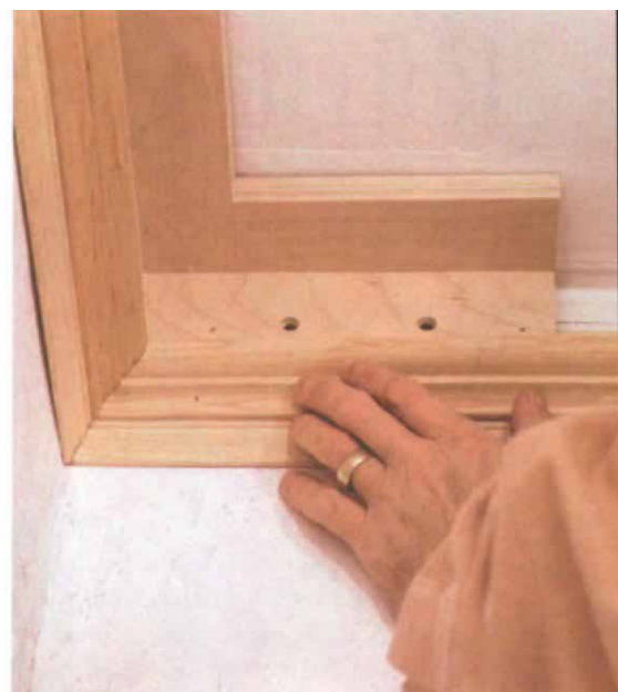
Coped joints are cleaner. The first two layers of this cornice, an inverted baseboard and a bed molding, were installed with coped joints at the inside corners.
